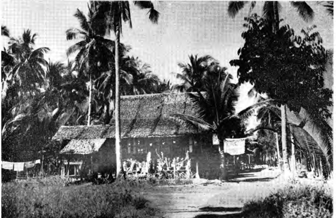
Fig. 3. A typical Malay house raised on stilts, with wooden floors and walls, and attap roof.
